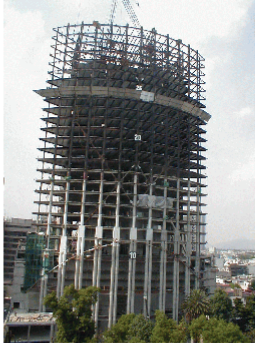
FIGURE 4 TORRE MAYOR BUILDING FRAME
