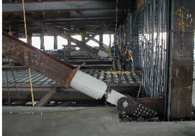
FIGURE 10 DAMPER INSTALLATION, SHORT WALLS
