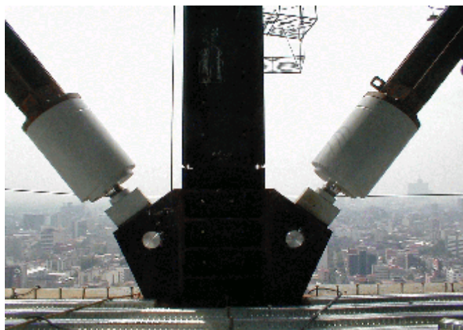
FIGURE 9 DAMPER INSTALLATION, LONG WALLS
