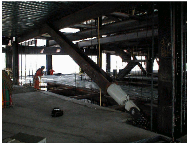
FIGURE 11 DAMPER INSTALLATION, SHORT WALLS
